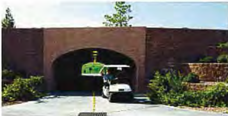
Figure 2-46A Hydro-Arch Cart Tunnel
